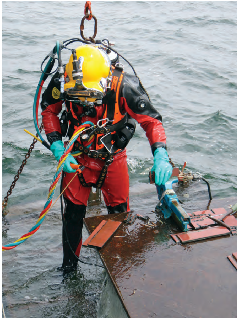
Fig. 9 — A fully equipped welder/diver preparing to go under for underwater welding and cutting. (Courtesy of Jan Hilkes.)
