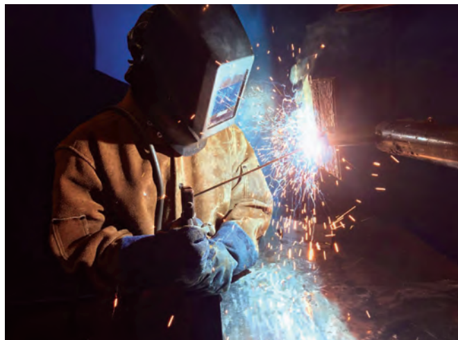
A welding student practices shielded metal arc welding in preparation for the 3G bend test. (Photo courtesy of Airport Community Schools.)
